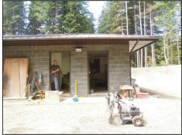
Figure 9. Water treatment building.
