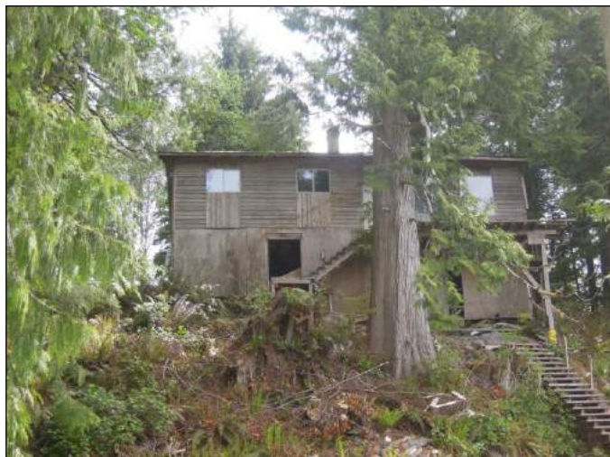
Figure 17. Residence with untreated wood siding, coniferous vegetation overhanging roof, and open decking which may trap embers. These factors greatly increase the fire hazard for this home.
