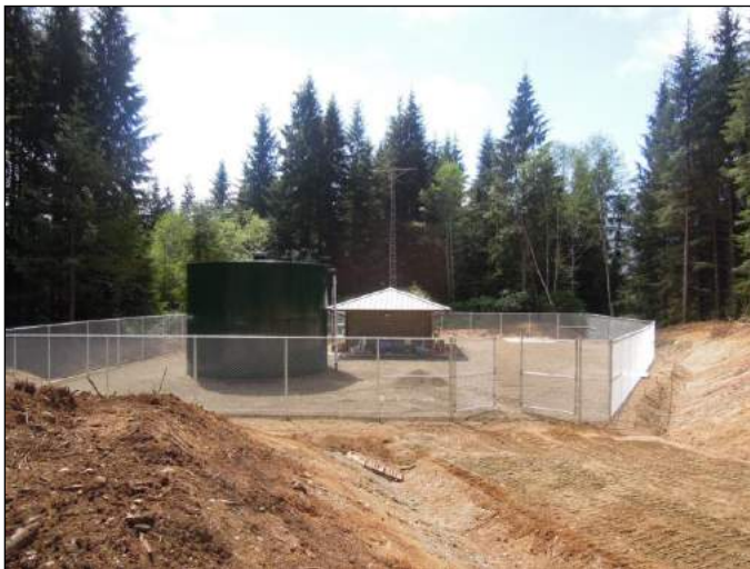
Figure 7. Water treatment building and reservoir.
