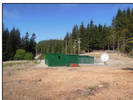
Figure 5. BC Hydro diesel generator.
