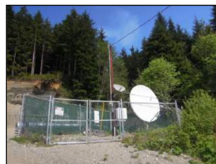
Figure 6. Monte Cristo Mountain Communications Tower
