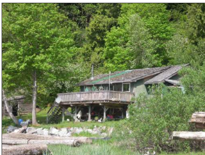
Figure 16. Combustible roofing (cedar shake) makes this house vulnerable to spotting. Deciduous and grass landscaping surrounding the home is low flammability which decreases the site hazard.
