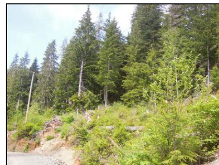
Figure 4. Transmission electrical infrastructure and right of way.
