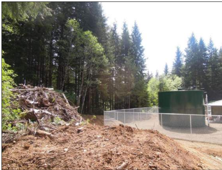
Figure 37. Slash accumulation as a result of clearing land for the water reservoir facility.
