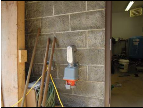
Figure 8. Emergency mobile generator hook-up in case of power outage at generating station.
